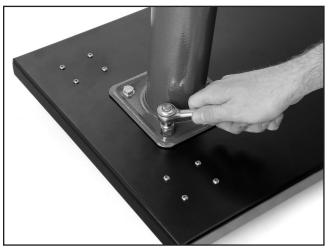
Figure 6. Installing collector support.
